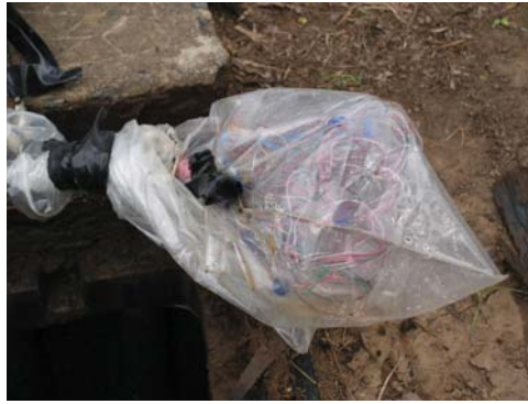
“Temporary” repairs. Note condensation inside bag.
